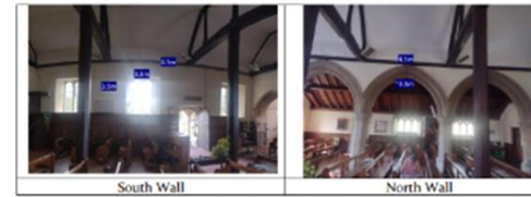
Photo 6: The Nave - showing the 3.5m and 4.5m heights. The central fire beams are 4.5m above the Nave floor.
