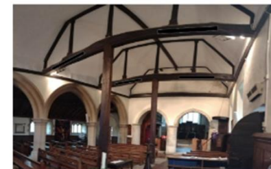
Photo 7: Nave showing mock-up of proposed Summit heating panels on central beams.
